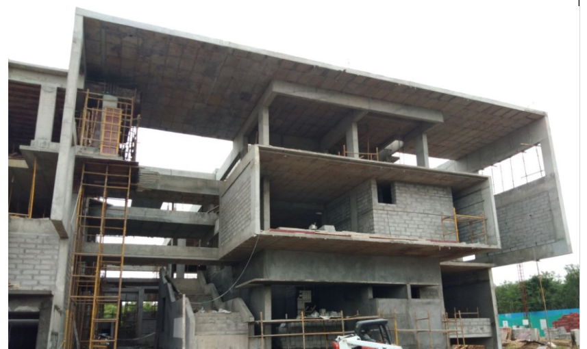
RCC Structural System
