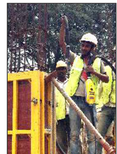
High Frequency Smart Poker 40MM - 12000 rpm 400 W
