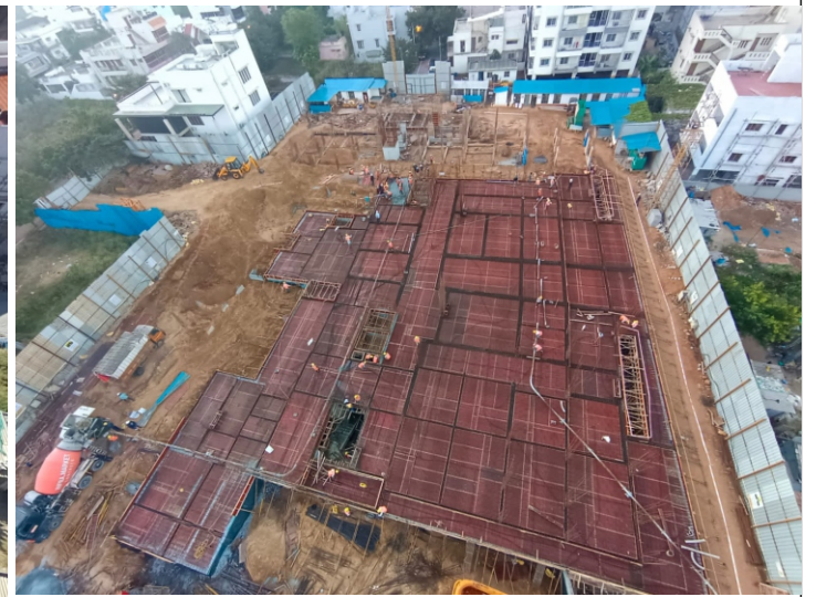
1st Slab Concrete
